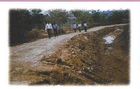
sunken ponds along rills interspersed with minipercolation tanks around ridge, a series of stone dams along gully to harvest soil, water trapping structures along the road ribbon and redirecting it to avenue trees through graded trenches were identified as some of the things to be done before arrival of rains. While the civil engineering wing is executing the works, the watershed faculty is covering the entire developmental process.
